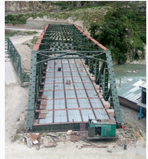
Steel Truss Bridge
