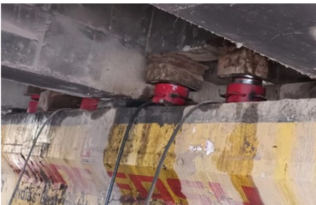
Lifting of RCC Bridge
