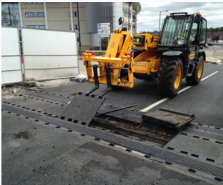
Expansion Joint Replacement
