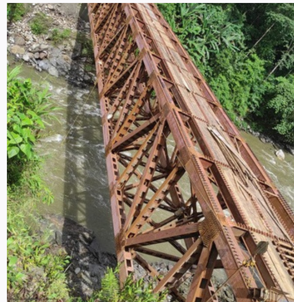
Deck Type Truss bridge
