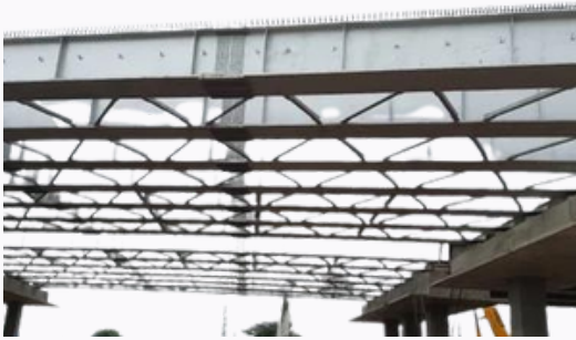
Steel Gider Bridge
