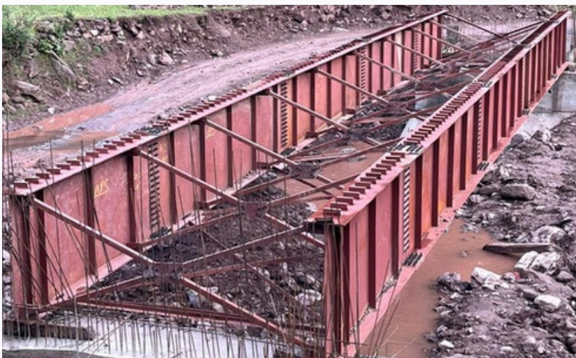
Plate Girder Bridge
